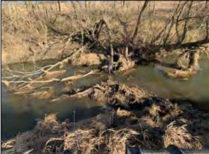
Downed tree removal east of CR 200 W - Wells Co.
